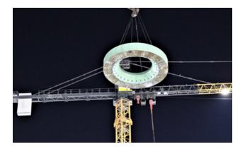
structure, which bears the load of the vessel, was assembled inside of the reactor pit. A week later, the third tier of the internal containment shell was installed, with quality of every weld confirmed by ultrasonic testing.
